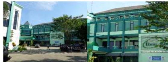
Figure 13: Application of the facade in the VIP Pavilion area.
