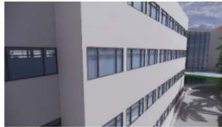
Figure 12: Existing Emergency Unit façade consist of walls, glasses window, and another opening.
