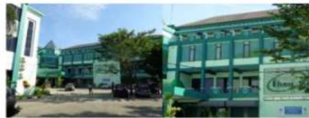
Figure 13: Application of the facade in the VIP Pavilion area.
